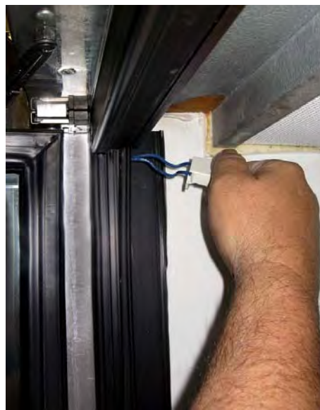
Step 4: Carefully remove both the top and bottom ELS sockets.
