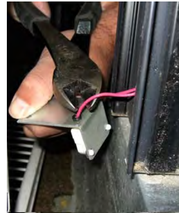
Step 4: Cut the socket power conductors.
