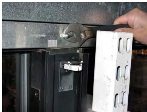
Step 5: Remove top raceway box nuts for the full length of the frame section.
