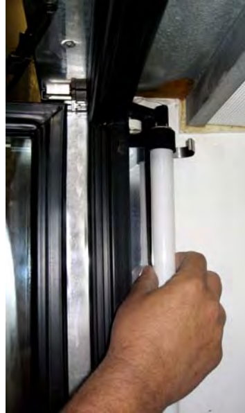
Step 2: Remove T-8 lamp from fixture.
